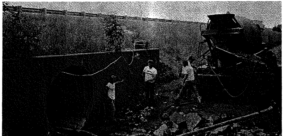
Figure 11 - An Ohio DOT rehab project. Concrete truck and pump in place on the downstream end of an 84 inch diameter Structural Plate Pipe under I-90.
