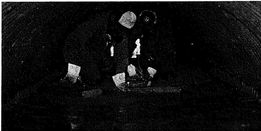
Figure 10 - Sealing the concrete pad surface inside a 58 inch x 36 inch Corrugated Steel Pipe-Arch in Jacksonville, OR.
