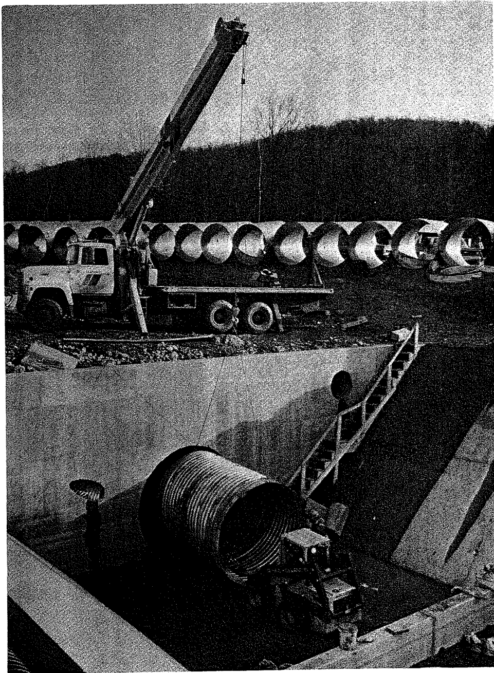
Figure 1 - A 96-inch dia. CSP being sliplined into a 108-inch dia. failed concrete pipe near Pittsburgh, PA.
